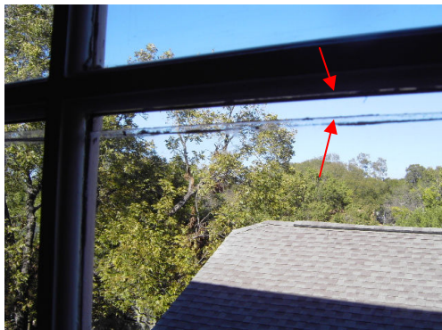
Photo of wood rot on outside of windows.
