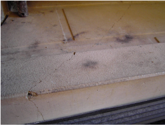
Please note cracked firebox above and approved hearth dimensions at right.
