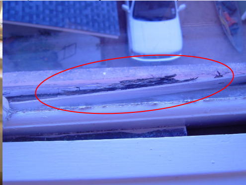
Photo of wood rot on outside of windows.
